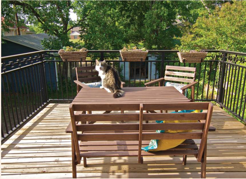
New balcony adds outdoor living space without increasing the home's footprint.
