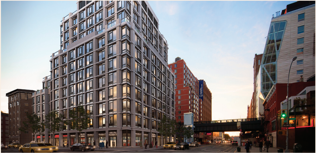
The façade of the TEN23 apartment building is a combination of poured-in-place ornamental concrete and sophisticated, highly insulated glass.
