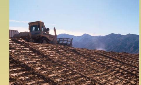
At the end of a working day, at least six inches of cover material is placed over the waste deposited that day. This helps to control litter and odors, and also compacts the waste.
