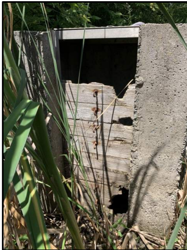
Photo 34: View of the stop logs present at the drawdown structure of Stormwater Pond 2. The logs have rotted and require replacement.
