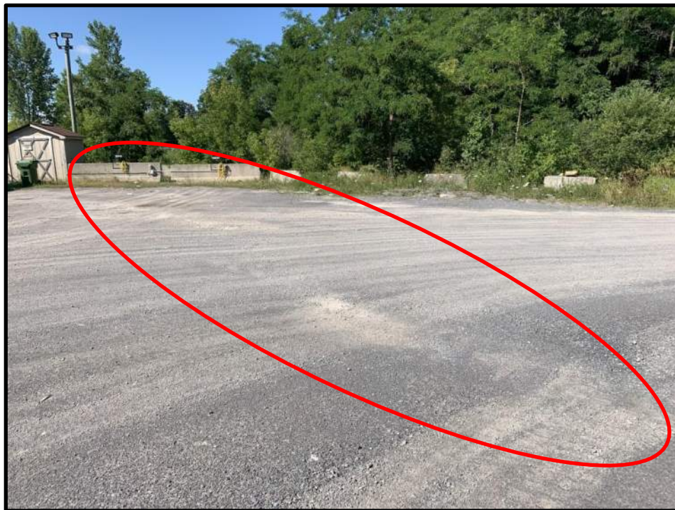
Photo 24: View facing west of a trench leading to the west side of the former public drop off facility southwest of the flare compound. Settlement of the trench (circled) has occurred, resulting in uneven road surface.
