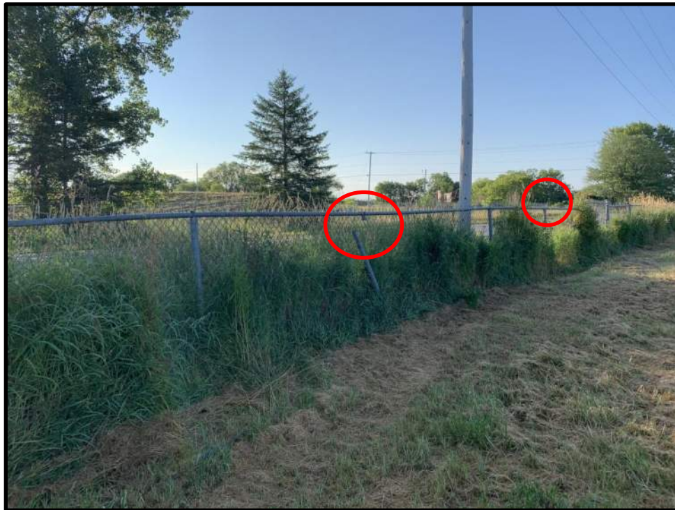
Photo 2: View facing southeast of the chain link fence along the east side of the landfill entrance. Some posts have separated from the top rail.
