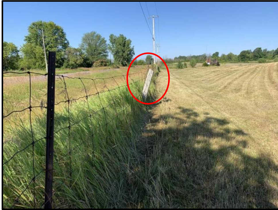
Photo 3: View facing west of a leaning fence post along the south perimeter of the site, east of the entrance. The paige wire has also dislodged from the post.
