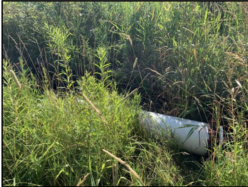
Photo 19: View of the outlet pipe at the west end of Stormwater Pond 3. The pipe is becoming obscured by vegetation.
