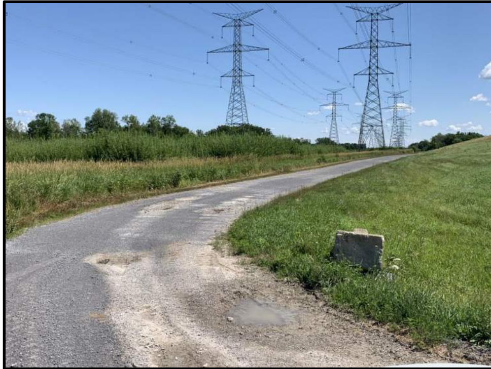
Photo 57: View facing northeast of standing water and potholes present in the surface of the northwest access road.
