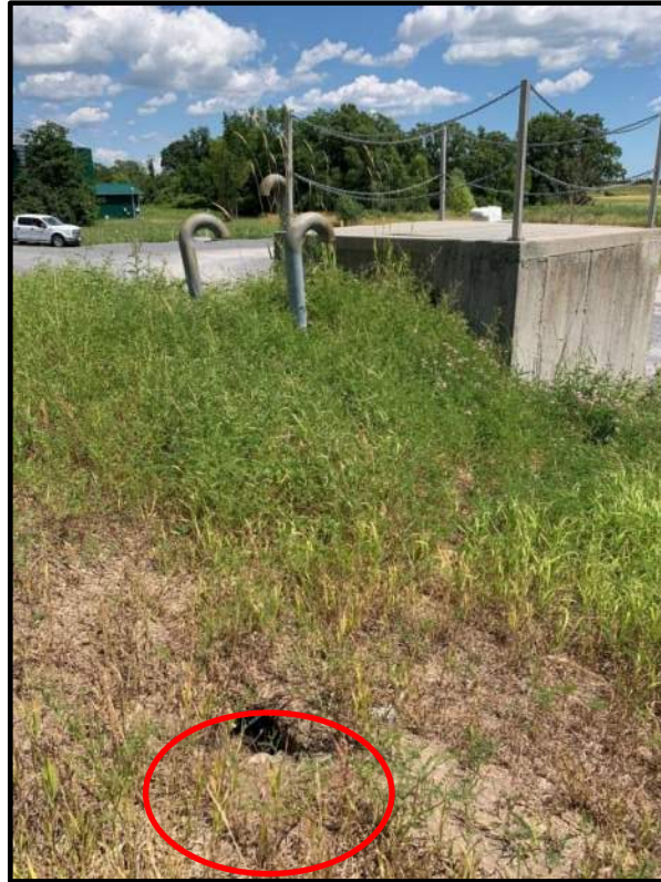
Photo 55: View facing southeast of the south slope with PS1 in the background. A hole (circled), potentially created by a rodent, is present in the area.
