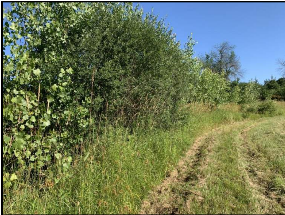
Photo 14: View facing north of the emergency spillway channel from Stormwater Pond 3. Thick vegetation is present in the channel.
