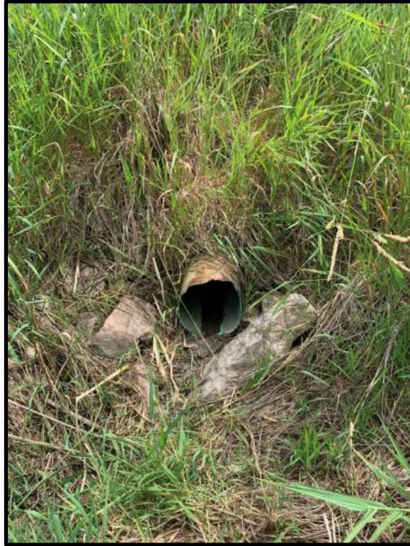
Photo 49: View of the outlet pipe from the drawdown structure at Stormwater Pond 1. No evidence of silt exiting the pond was observed.
