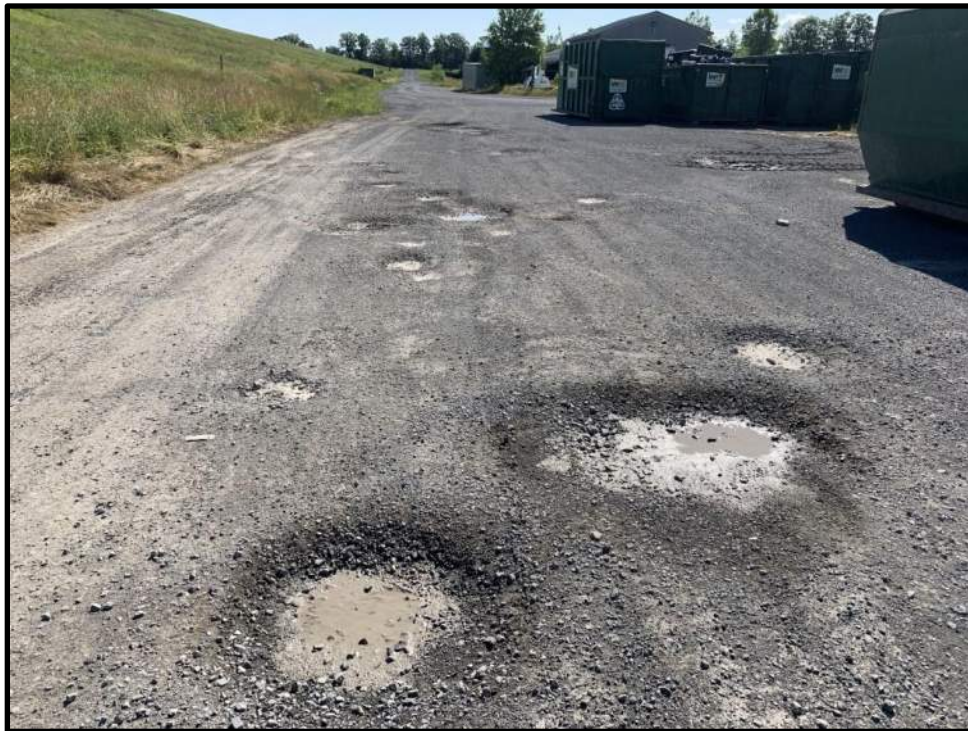
Photo 26: View facing east of the south perimeter road, east of the flare compound. Several roll off bins are present at the tee intersection, which limits sight line for oncoming traffic. Several large potholes are also present in the road surface.
