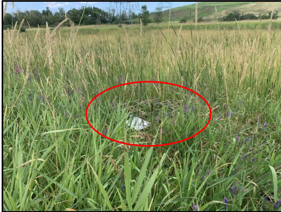
Photo 47: View of the drop inlet pipe structure (circled) at Stormwater Pond 1. Vegetation has obscured the structure.
