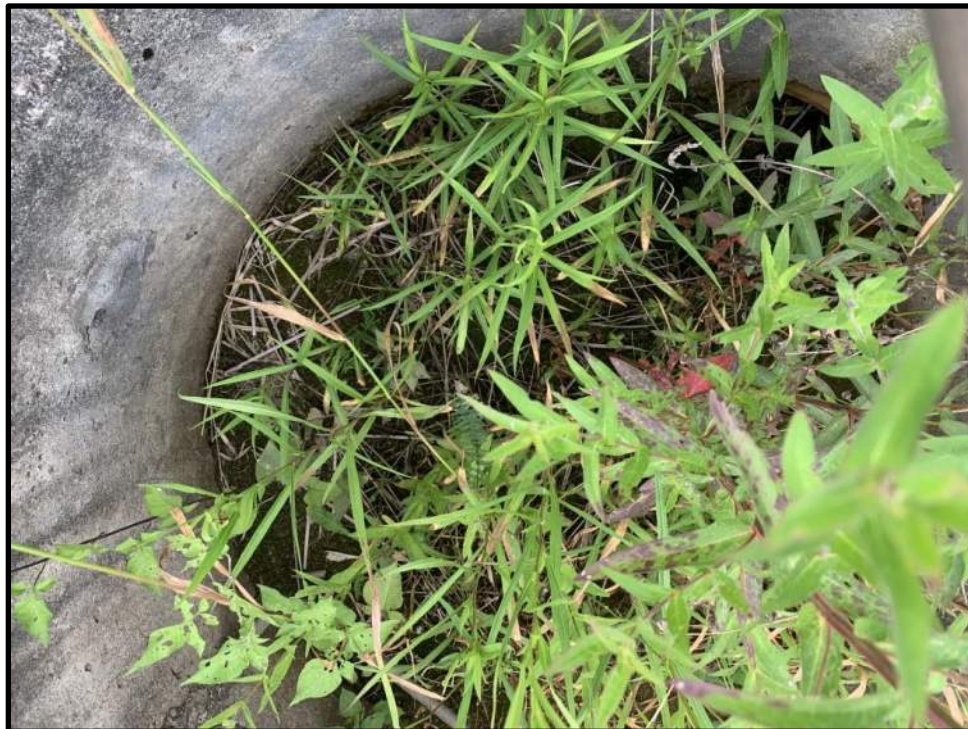
Photo 48: View looking down into the drop inlet structure at Stormwater Pond 1. The inlet pipe can be seen on the upper right side of the photo. The pipe is partially obscured by vegetation and sediment.
