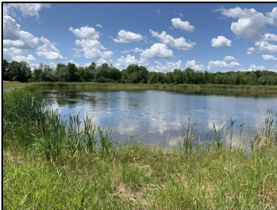
Photo 40: View facing west of the leachate holding lagoon. No evidence of rodents (no damage to the HDPE liner) was observed. Debris observed in the southeast corner of the lagoon during a previous inspection was not seen during this visit.
