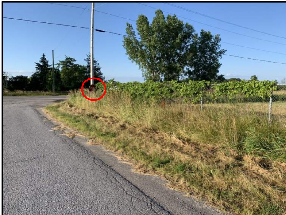
Photo 6: View facing southwest of the Stop sign at the landfill entrance. The Stop sign is leaning away from the traffic sight line and thick vegetation is obscuring the emergency evacuation signage on the fence.
