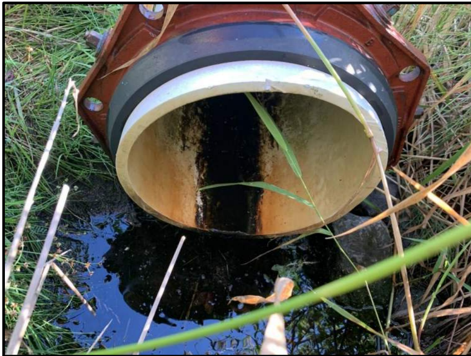
Photo 20: View of the outlet pipe to the emergency spillway channel at Stormwater Pond 3. A small pool of water is present under the pipe.
