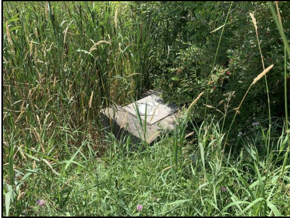
Photo 35: View of the drawdown structure at Stormwater Pond 2. Vegetation has obscured the ground at the structure, preventing observations of the access path to the structure.
