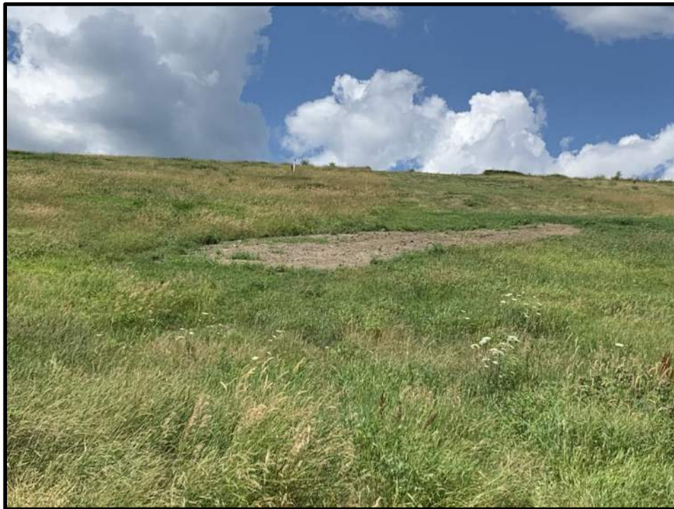
Photo 52: View facing north of a seep repair on the south slope of the landfill mound. The repair was completed by a subcontractor to WM in May 2022. Vegetation has yet to establish in the area.
