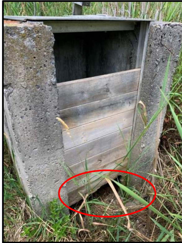
Photo 45: View of the stop logs on the draw down structure at Stormwater Pond 1. Boards at the base of the structure have rotted and require replacement.
