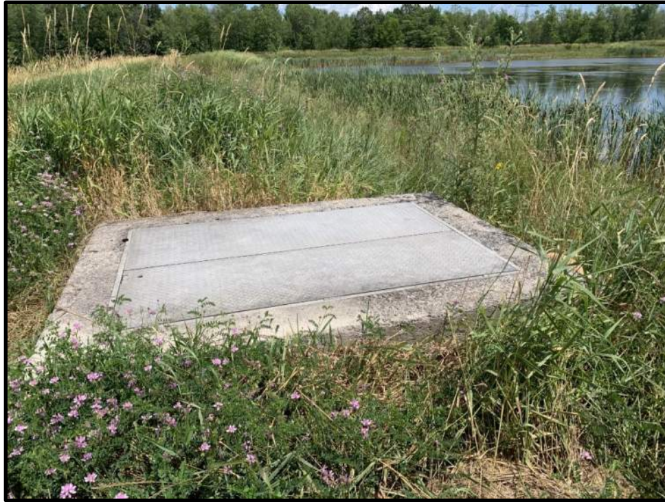
Photo 41: View facing east of the northwest structure at the leachate holding lagoon. “Confined Space” signage was not observed.
