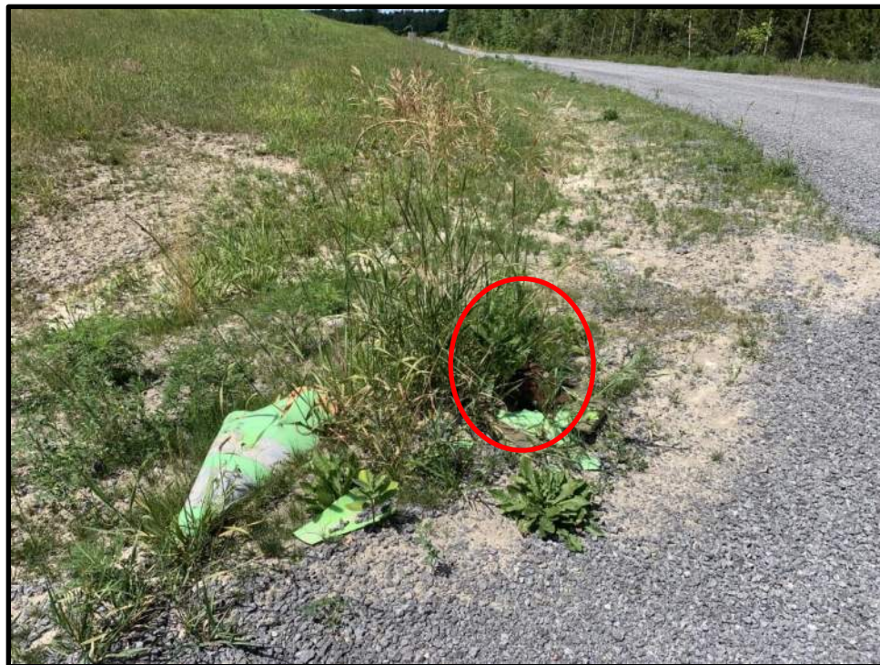
Photo 56: View (encircled) of damage to monitoring well M19 on the southeast corner of the landfill. It is not clear if the well is part of the site's monitoring network.
