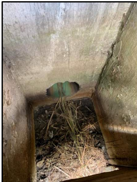
Photo 46: View of the interior of the drawdown structure at Stormwater Pond 1. The inlet is free of sediment.
