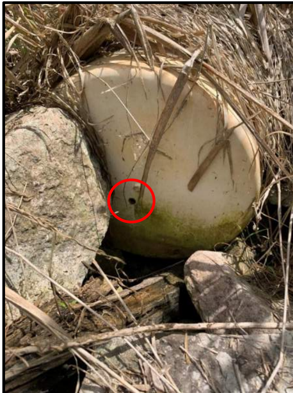
Photo 50: View of the outlet pipe from the drop inlet pipe structure at Stormwater Pond 1. A cap is present on the outlet pipe, but a small hole in the cap was noted (circled).
