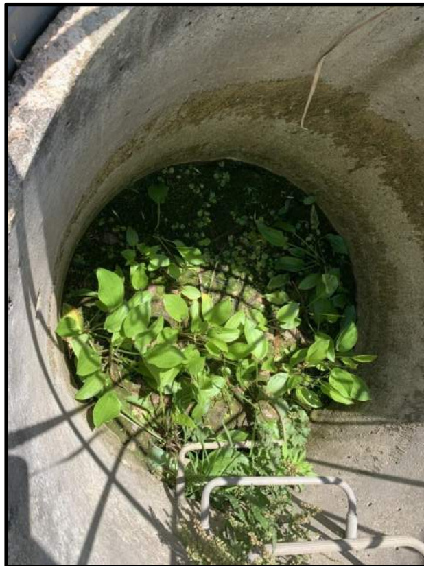
Photo 38: View inside drop inlet pipe structure at Stormwater Pond 2. Sediment is present in the structure along with vegetation. The outlet pipe (under the rungs) is not visible.
