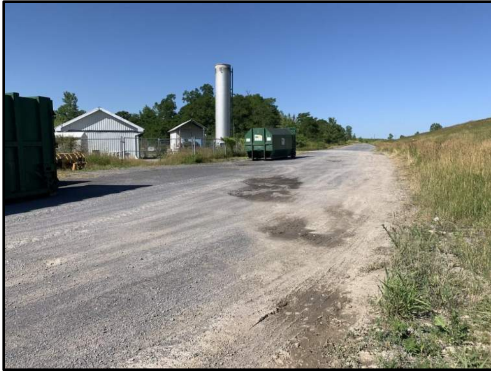
Photo 23: View facing west of the south access road east of the flare compound. The trench containing the electrical cable from PS3 near the leachate storage tank has experienced settlement and potholes are visible.
