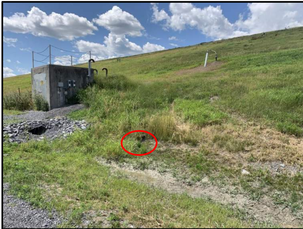
Photo 54: View facing northwest of a small section of staining (circled) present at the top of the south ditch east of PS1. A small amount of water is present in the ditch below the stained area.
