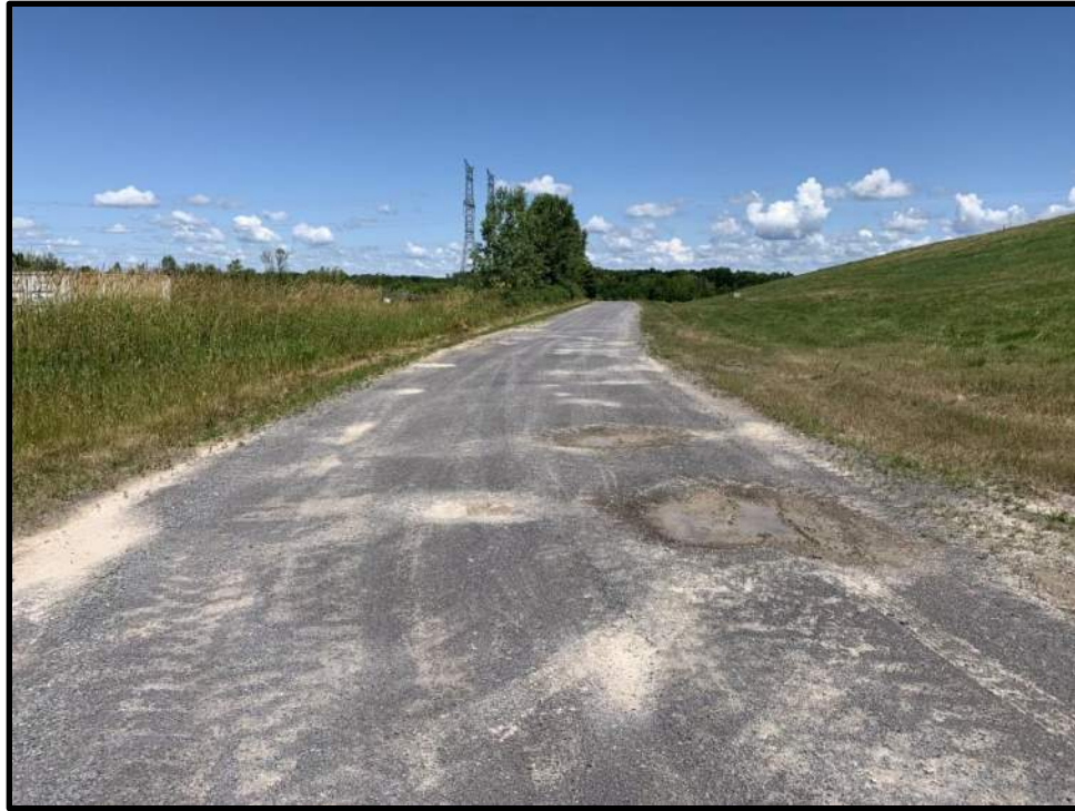
Photo 59: View facing north of several potholes along the southwest perimeter access road.
