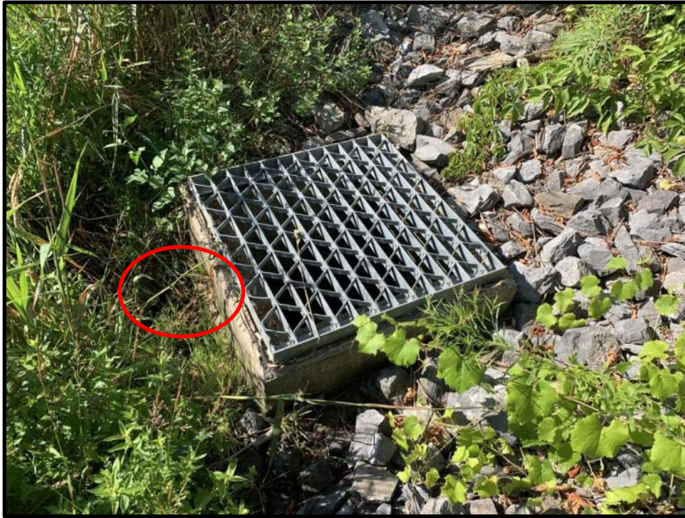
Photo 17: View of the inlet structure on the west side of Stormwater Pond 3, east of the emergency spillway. Vegetation is surrounding the inlet side of the structure (circled) but water can still enter the inlet.
