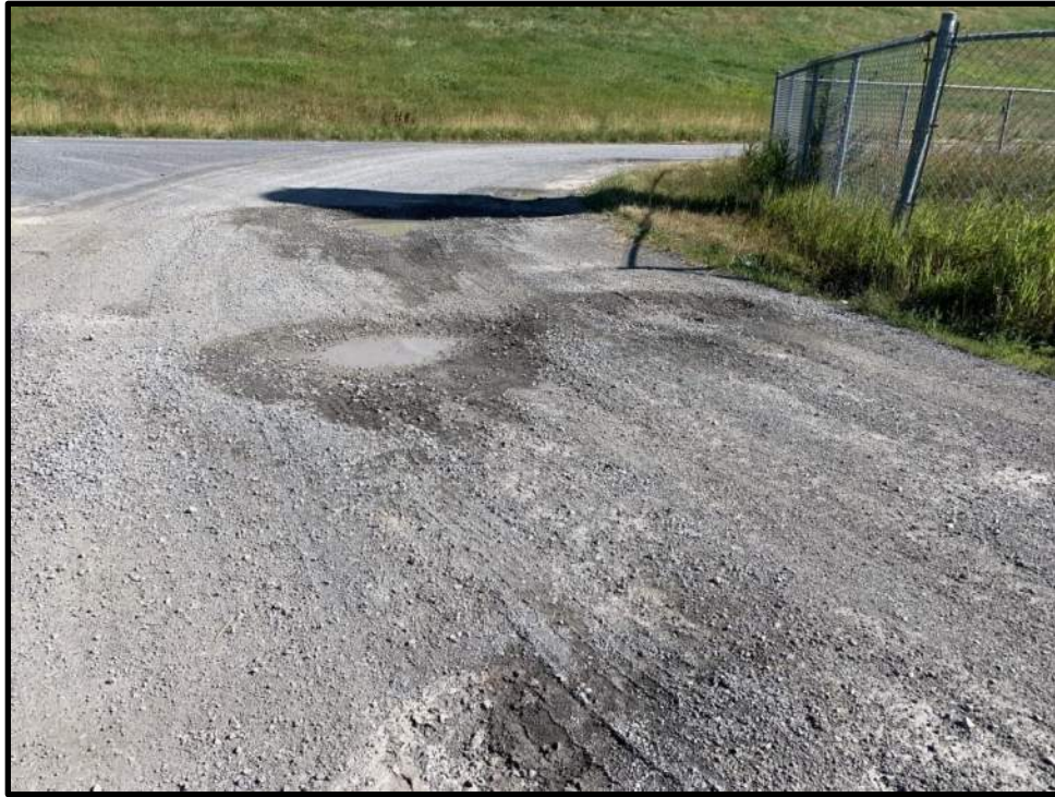
Photo 25: View facing north of several deep potholes present in the road surface to the west of the flare compound.
