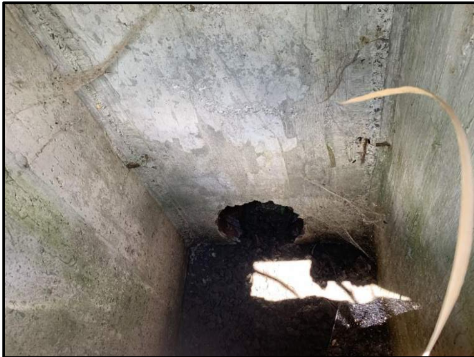
Photo 36: View inside the drawdown structure at Stormwater Pond 2. The inlet pipe is free of debris.
