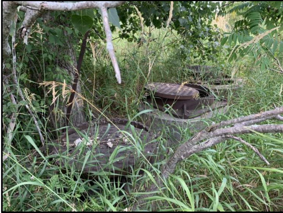
Photo 61: View facing south of dislodged lids at the interceptor chamber south of the former contaminated soil pad. No “Confined Space” signage is present.
