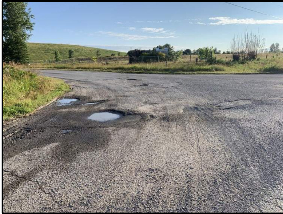
Photo 1: View facing north of the pavement at the site entrance off Beechwood Road. Potholes are emerging on the southwest portion of the road.
