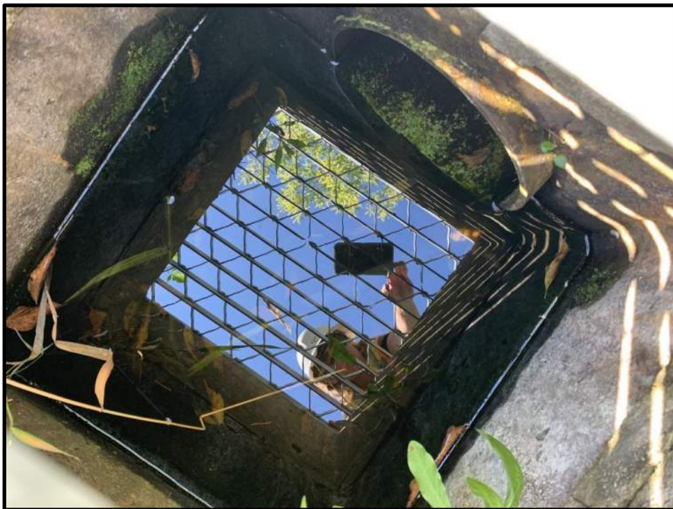
Photo 18: View inside the inlet structure at Stormwater Pond 3, east of the emergency spillway. Water can freely exit the structure once levels are high enough.
