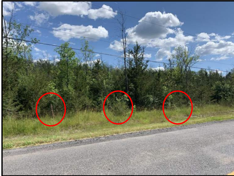
Photo 7: View facing southwest of a section of the north perimeter fence along Selby Road, east of the former Wildlife Habitat house. Fence posts in the area are leaning or are missing; the paige wire fence is down; and the “No Trespassing” signs are not present in this location
