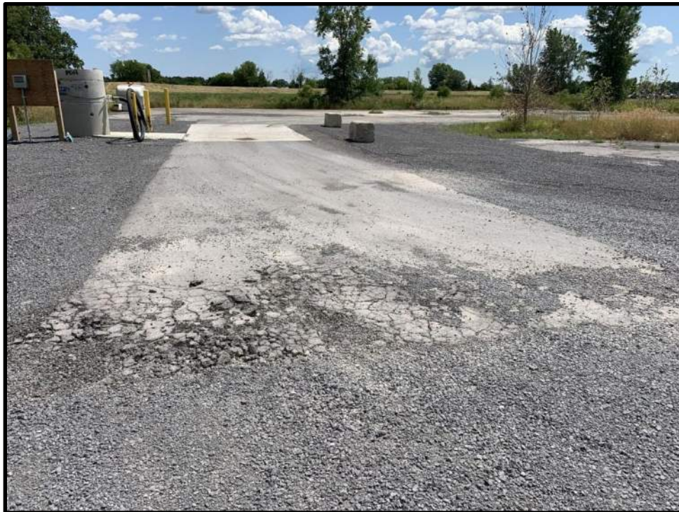
Photo 62: View facing south of the north side of the asphalt at the leachate storage Tank loading area on the east side of the former contaminated soil pad. The asphalt is displaying signs of wear.
