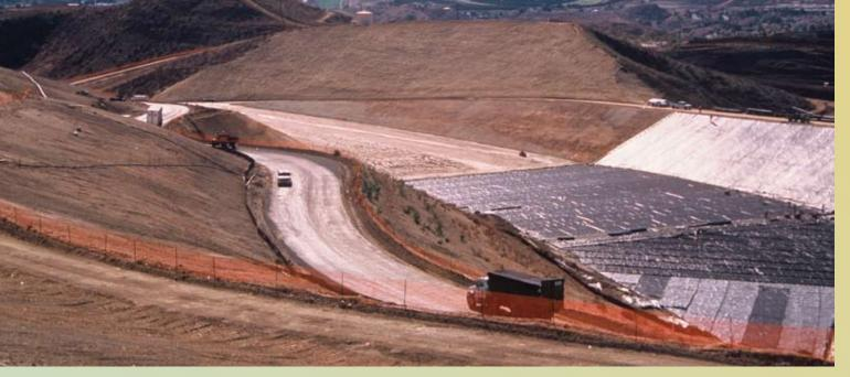
in the landfill and compacted. The landfill's liner and gas and leachate extraction systems protect the surrounding land and water supply, and operating procedures include regular environmental monitoring.
