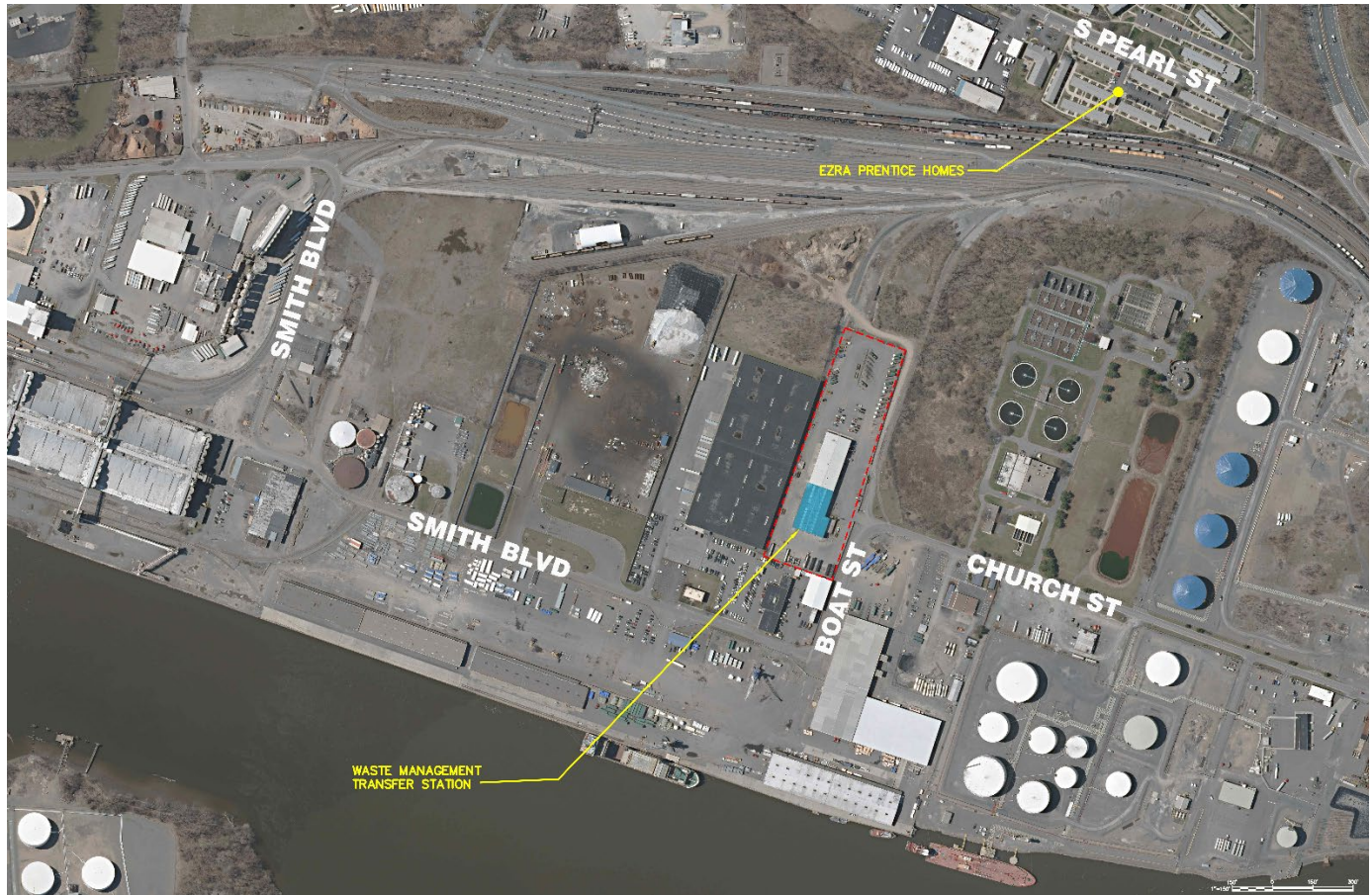
Aerial Image Port of Albany Transfer Station operated by Waste Management of New York, Inc., 100 Boat Street.
