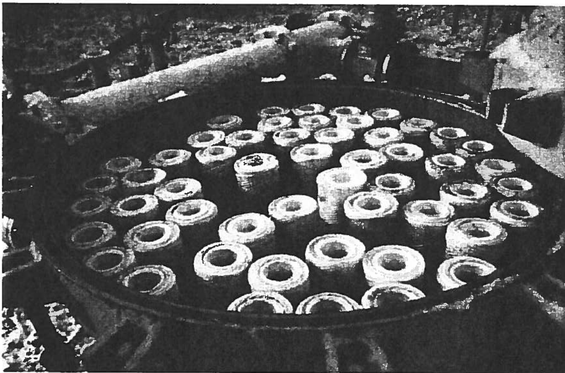
Photo #4 - Photo of Effluent Disharge System Filtration Media Cartridges.
