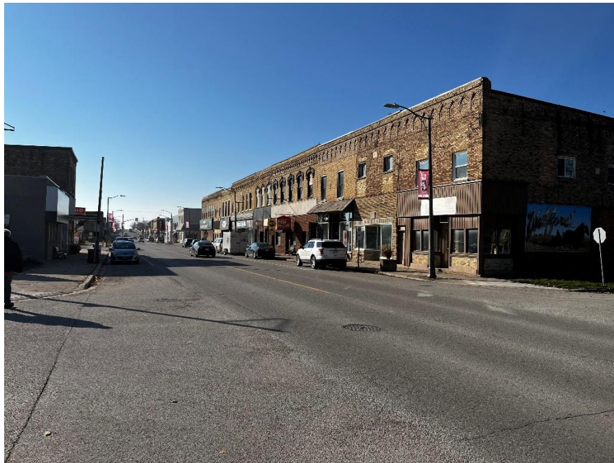
Figure 5-13. Watford Village commercial centre, looking southwest on Nauvoo Road
