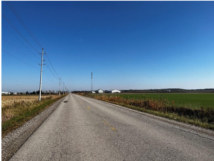
Figure 5-1. Zion Line, looking east toward the intersection with Nauvoo Road
