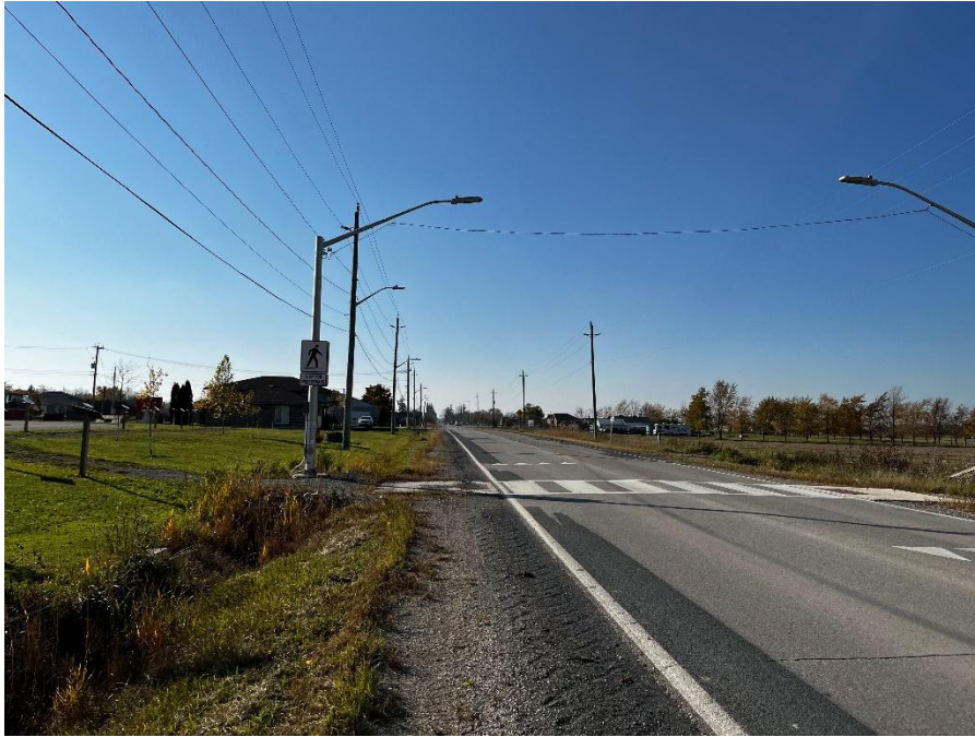
Figure 5-11. Confederation Line, looking west
