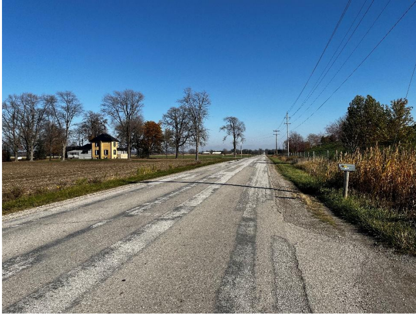
Image 1: Area has been previously assessed, no potential.
