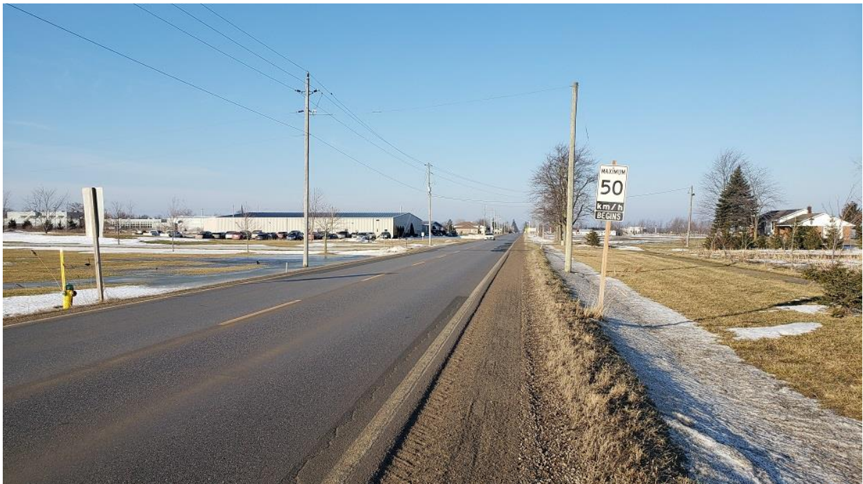
Confederation Line – Looking West – Approximately 700 metres east of Nauvoo Road
