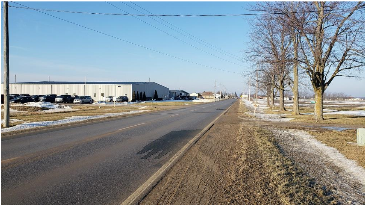
Confederation Line – Looking West – Approximately 640 metres east of Nauvoo Road
