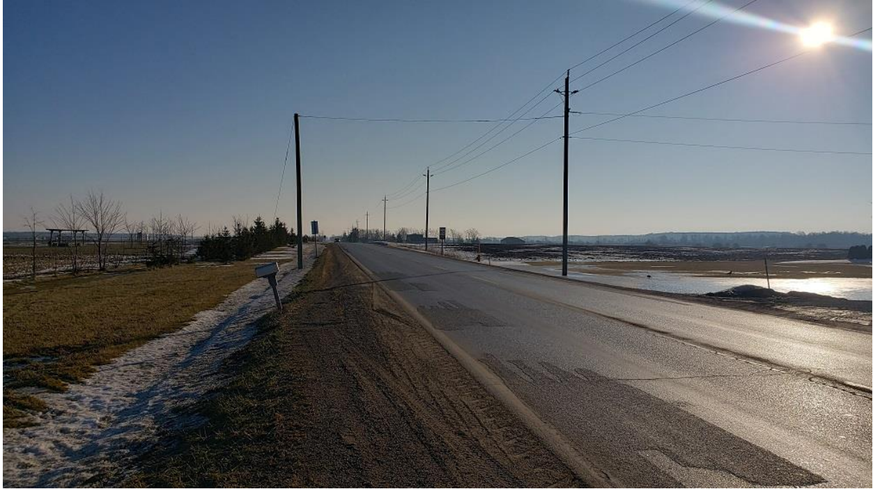
Confederation Line – Looking East – Approximately 640 metres east of Nauvoo Road
