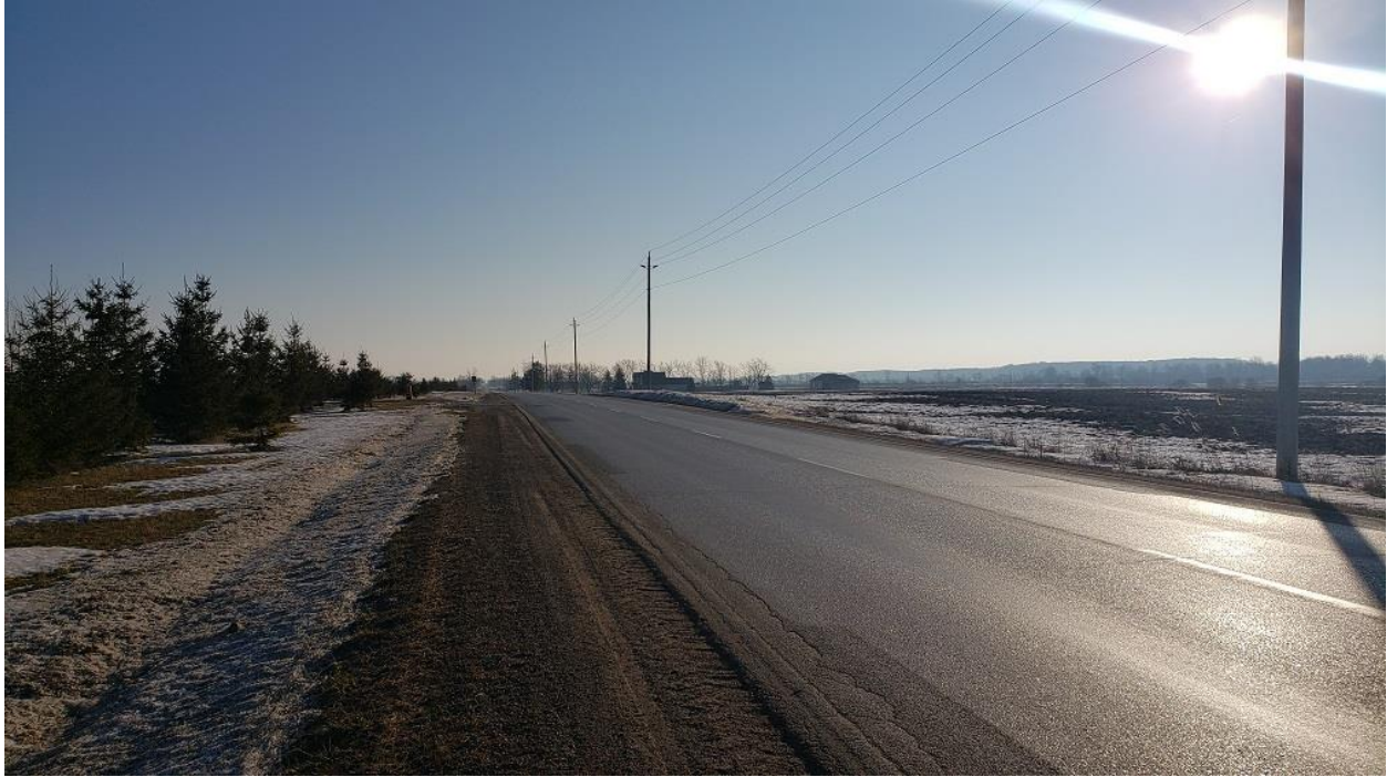
Confederation Line – Looking East – Approximately 700 metres east of Nauvoo Road
