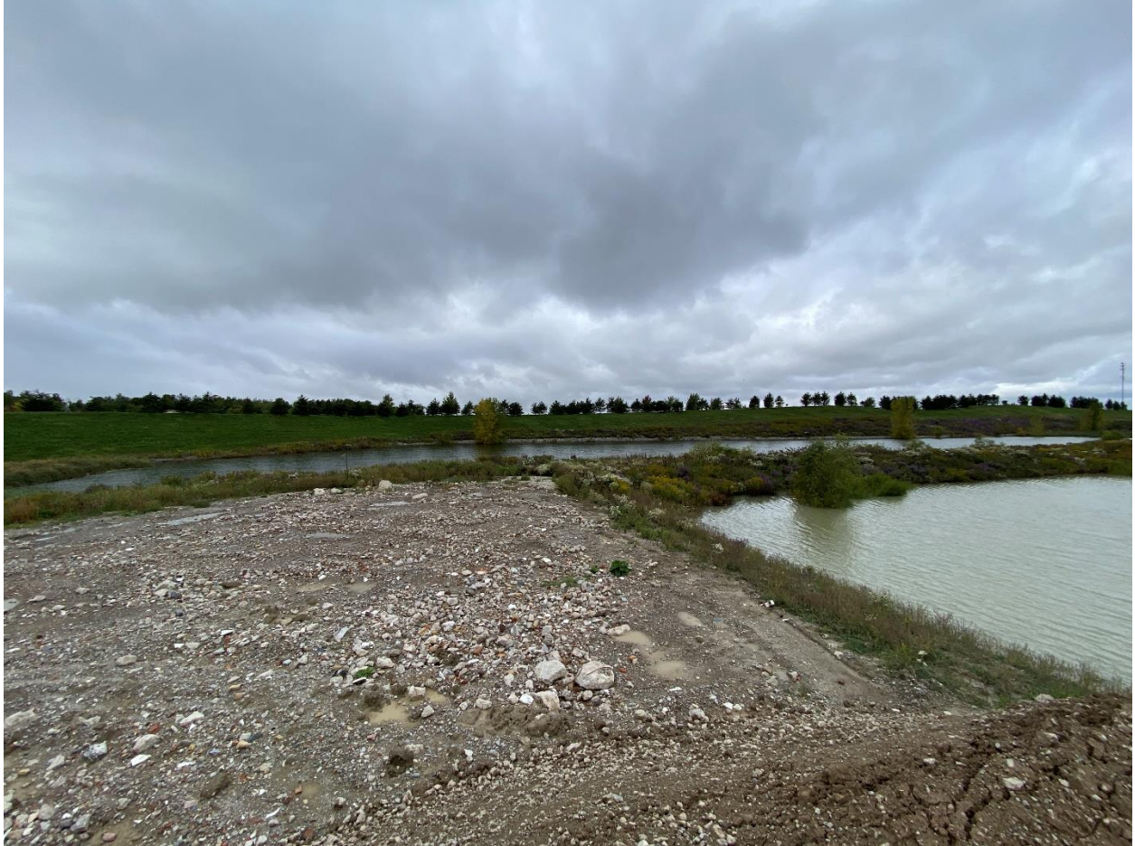
Image looking north shows the forebay and the berm that divides the forebay and the main cell of the SWM pond.
