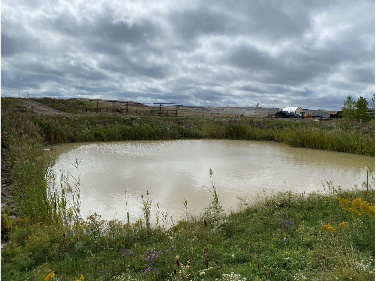
SWM Pond 4 located in the northeast corner of the site. Image looking southwest towards the site with the forebay shown in foreground.
