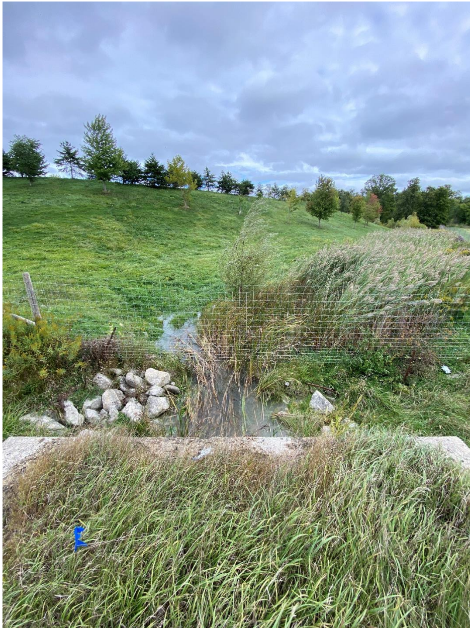
Nauvoo Road culvert looking east (upstream) towards the site.
