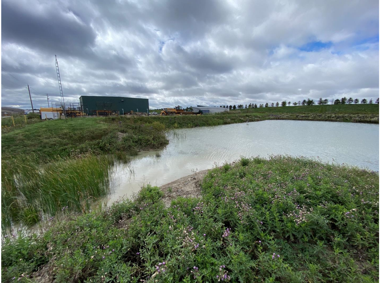
Image looking southwest shows the SWM pond forebay in foreground.
