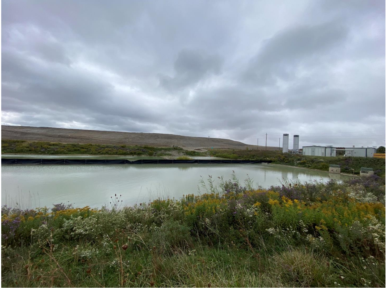
Looking west towards the RNG facility near SWM Pond 1.
