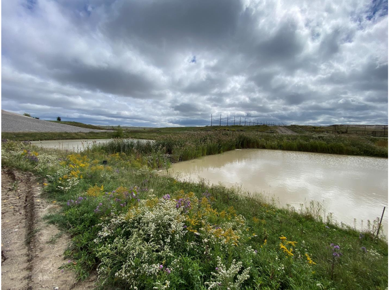
Image looking south shows the forebay in foreground and the main cell in distance.
