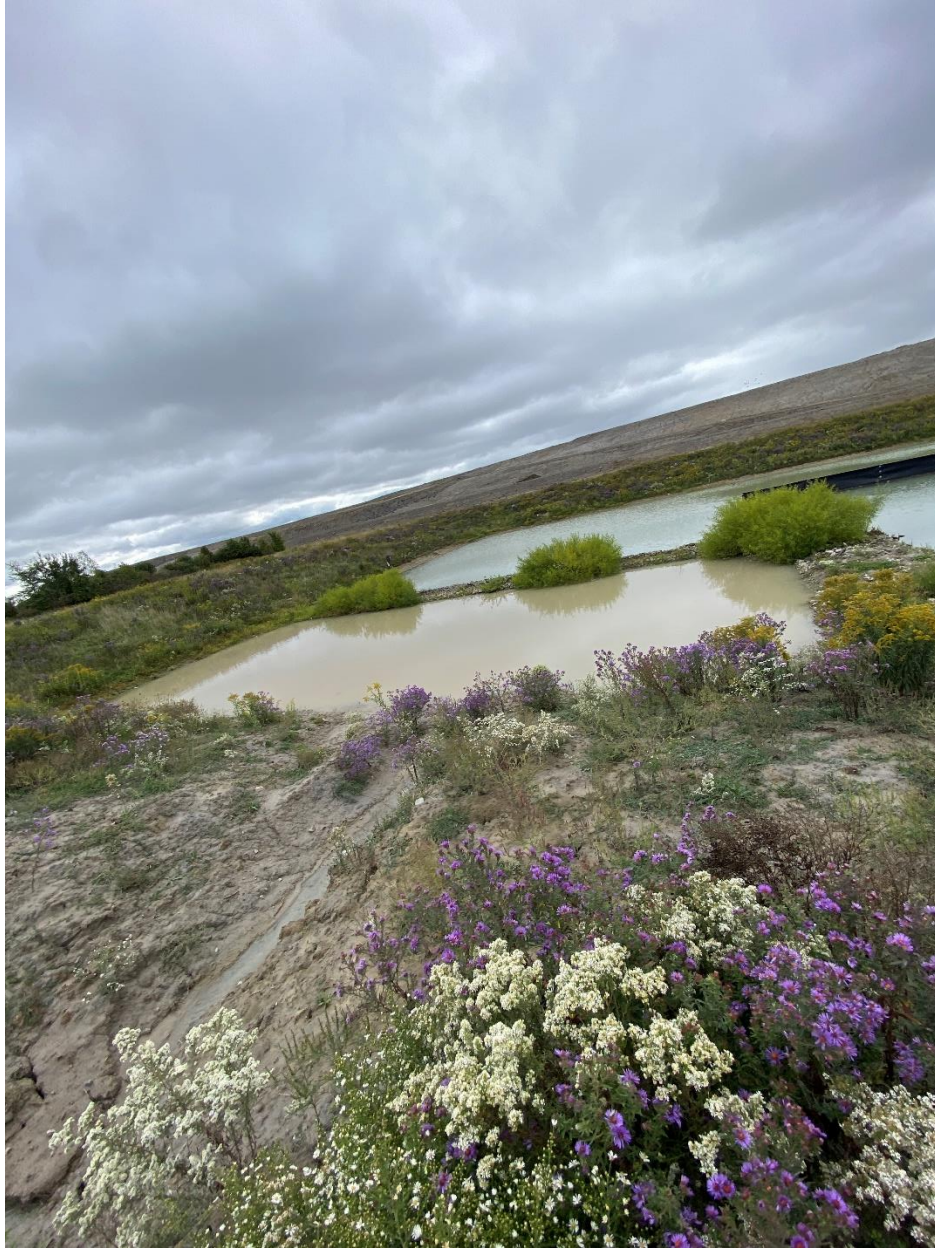
Inflows entering the forebay of the SWM Pond 1 from the South Cell of the site near Street 'E' overlooking the forebay that is separated from the main cell by a berm.
