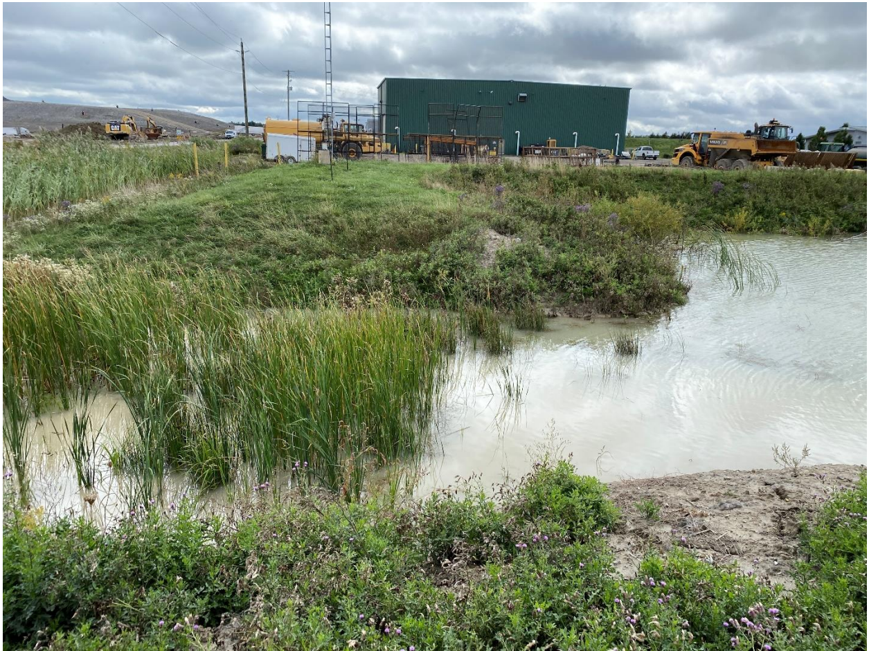
SWM Pond 3 located in the southwest corner of the site. Image looking south towards the maintenance building shows inflows into the pond.
