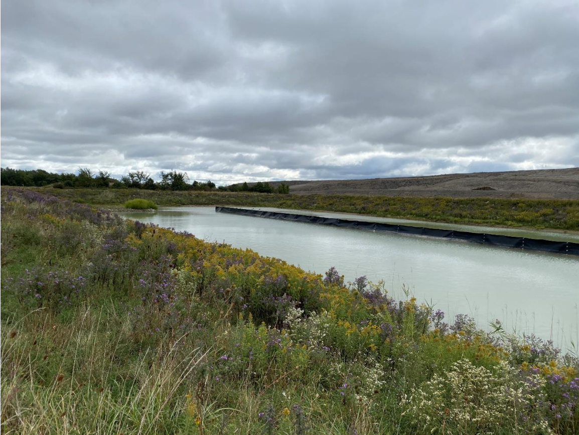
SWM Pond 1 located at the southeast corner of the site. This image is overlooking the main cell of the pond towards east.
