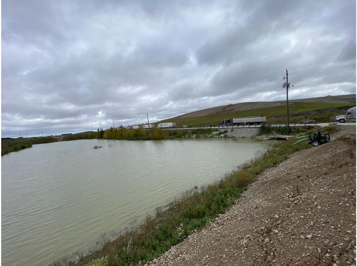
Image looking east shows the forebay and Street 'C' in distance.
