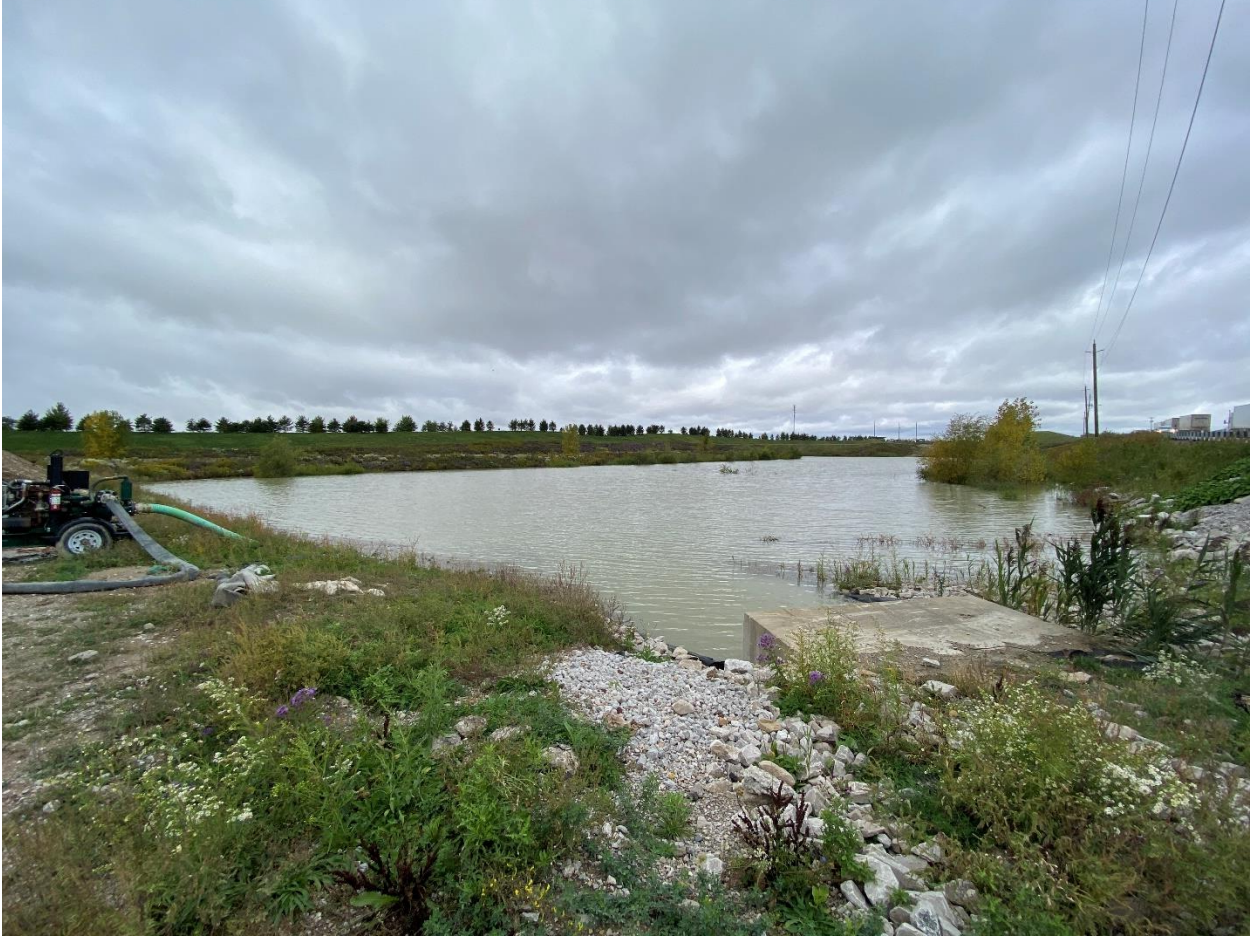
Image looking west shows inflows into the pond from the reinforced concrete box culvert near Street 'C'.
