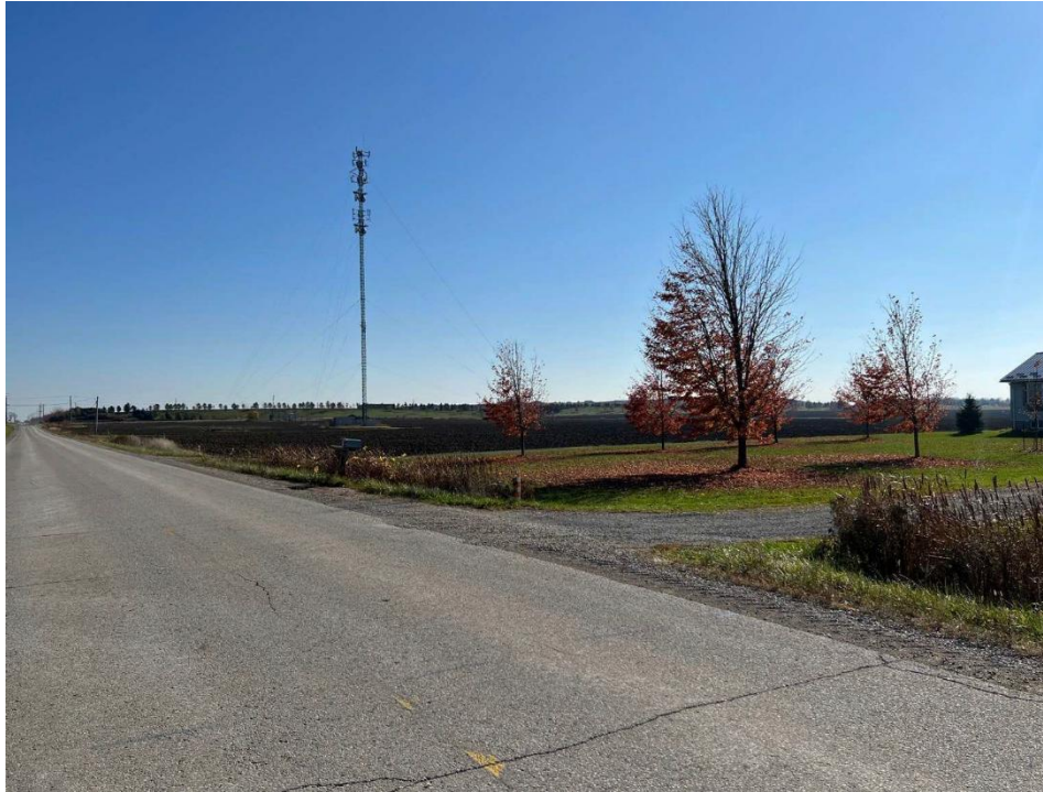
Photo 32 - Zion Line west of Nauvoo Road viewing E / SE
