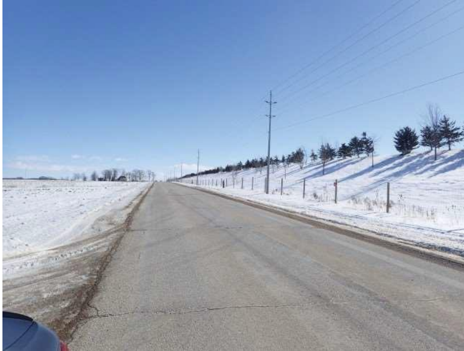
Photo 24 - Zion Line west of Nauvoo Road viewing east
