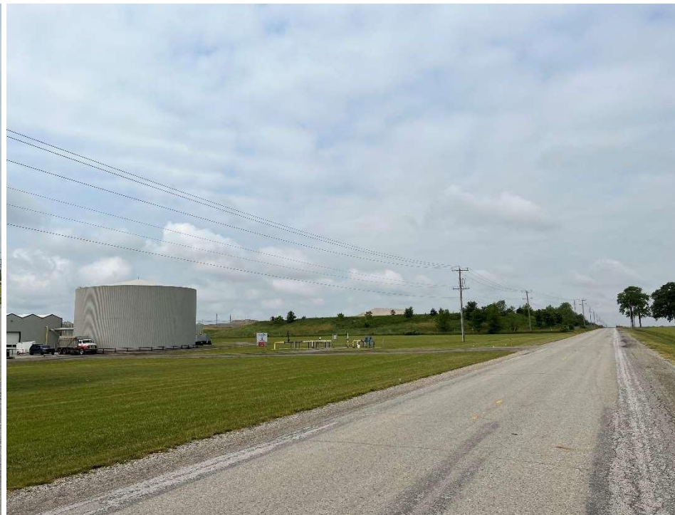
Photo 23 - Zion Line viewing S/W to Twin Creeks Greenhouse Complex at N/E corner of Twin Creeks Environmental Centre
