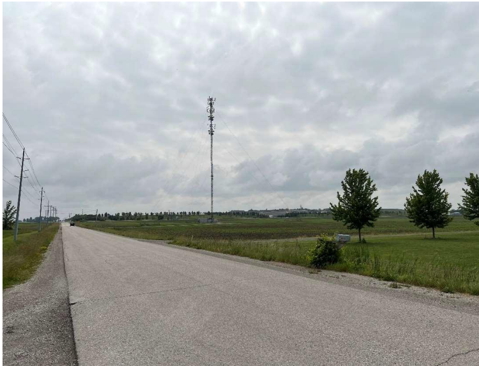
Photo 31 - Zion Line west of Nauvoo Road viewing E / SE
