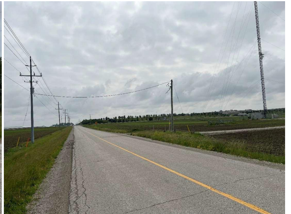
Photo 30 - Zion Line west of Nauvoo Road viewing east
