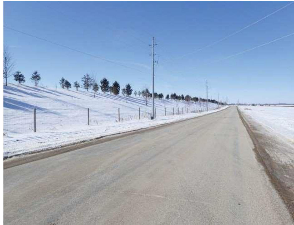
Photo 26 - Zion Line west of Nauvoo Road viewing east
