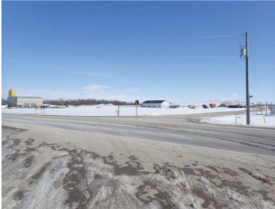
Photo 44 - West side of Nauvoo Road 0.7km north of Confederation Line viewing N/E
