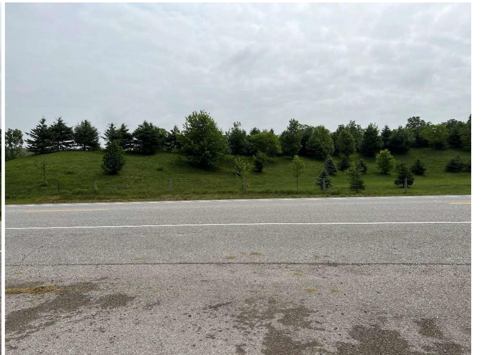
Photo 42 - West side of Nauvoo Road viewing east
