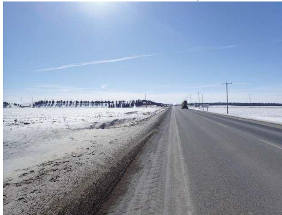
Photo 29 - Nauvoo Road north of Zion Line viewing S/SE and south
