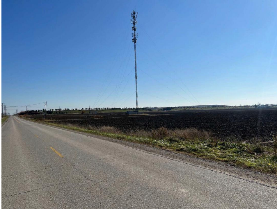
Photo 31 - Zion Line west of Nauvoo Road viewing E / SE
