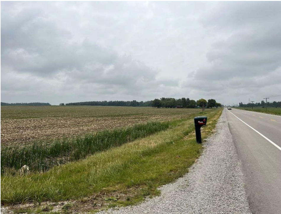
Photo 62 - Viewing south from east side of Nauvoo Road, north of Highway 402
