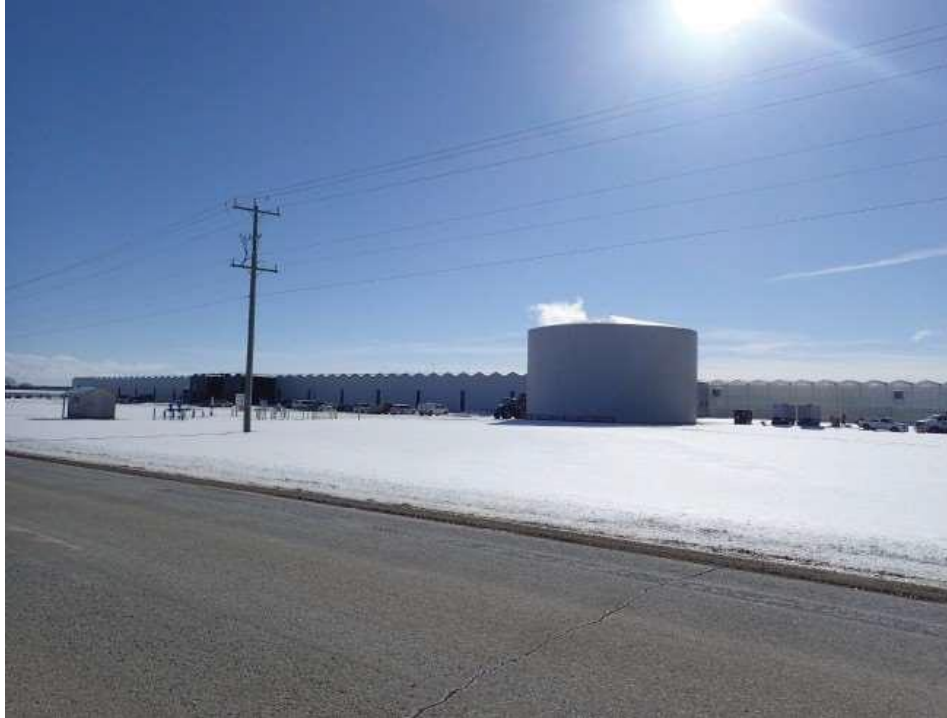
Photo 23 - Zion Line viewing S/W to Twin Creeks Greenhouse Complex at N/E corner of Twin Creeks Environmental Centre
