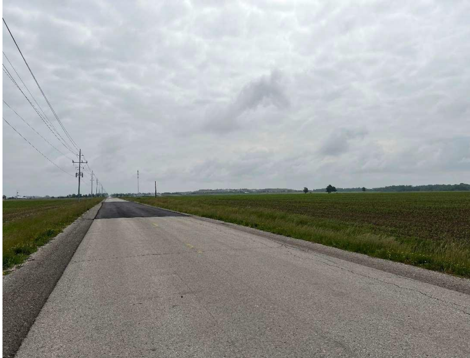
Photo 34 - Zion Line east of Underpass Road viewing E / SE
