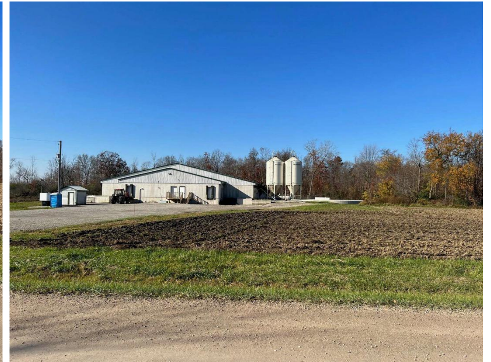
Photo 15 - View westward from Arkona Road between Confederation Line and Zion Line
