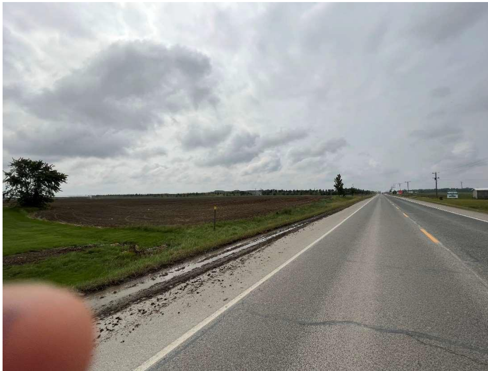
Photo 28 - Nauvoo Road north of Zion Line viewing S/SE and south
