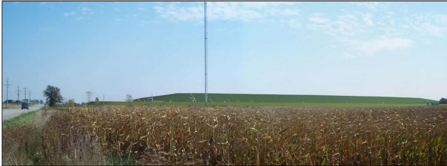
FROM ZION LINE VIEWING EAST
