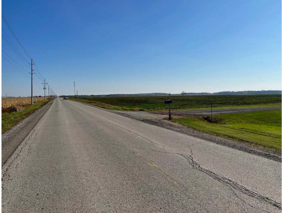
Photo 34 - Zion Line east of Underpass Road viewing E / SE
