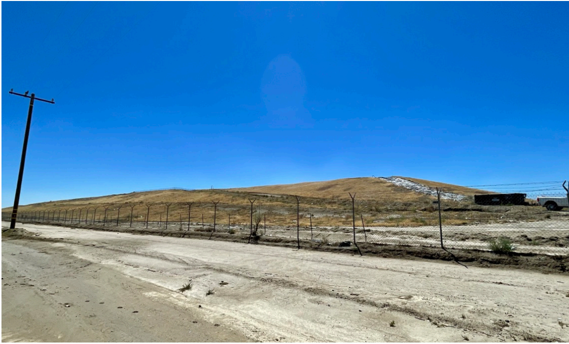
Photograph 3. Looking east along Ave F, at the west end of the north slope.
