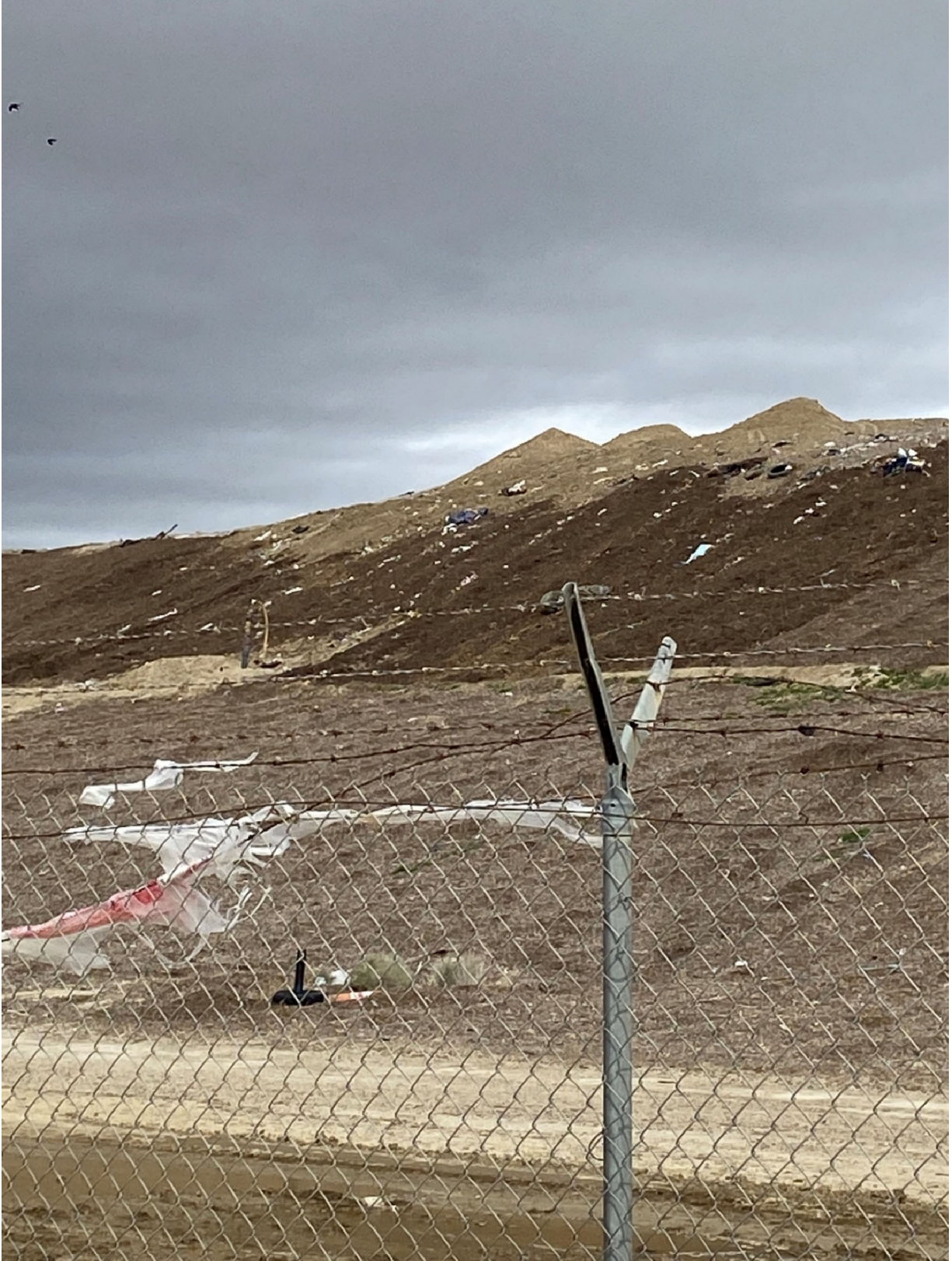
Photo 6: Refuse uncovered blown onto mulch interim cover southeast portion of site.
