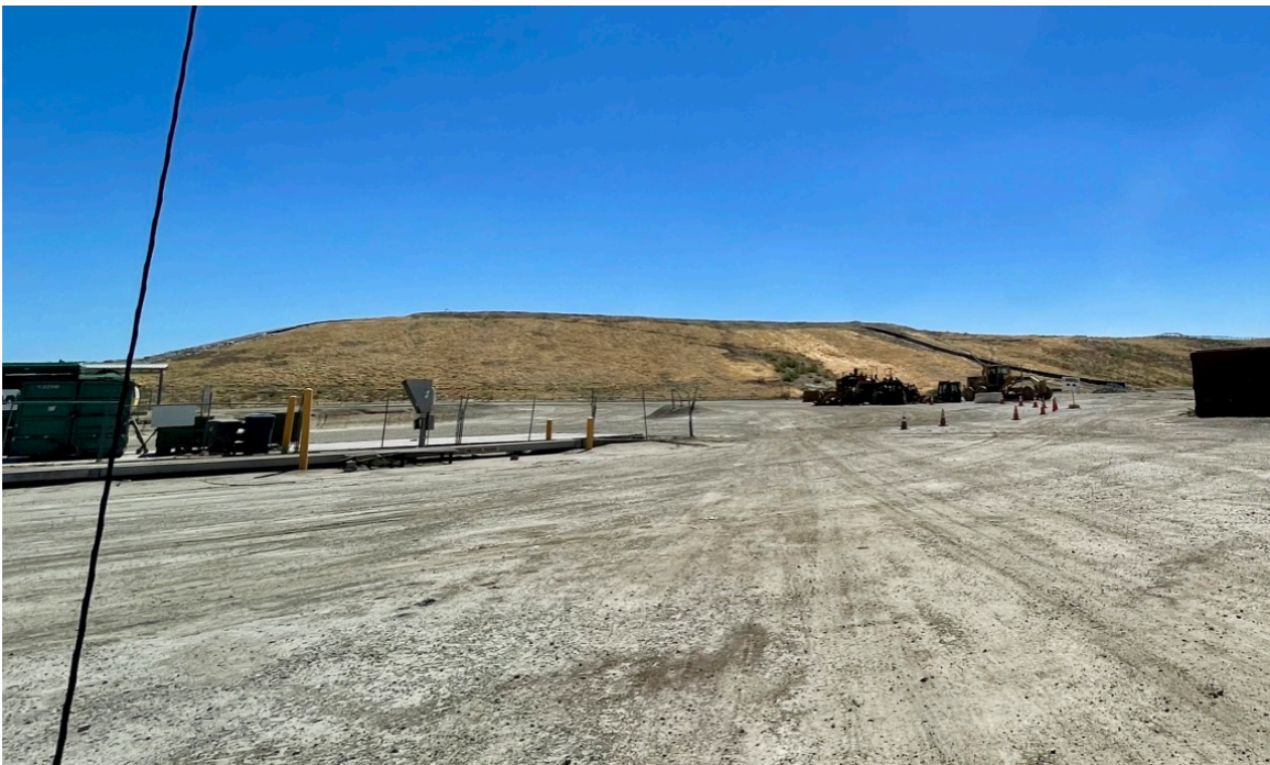
Photograph 2. The west facing temporary slope near the office.
