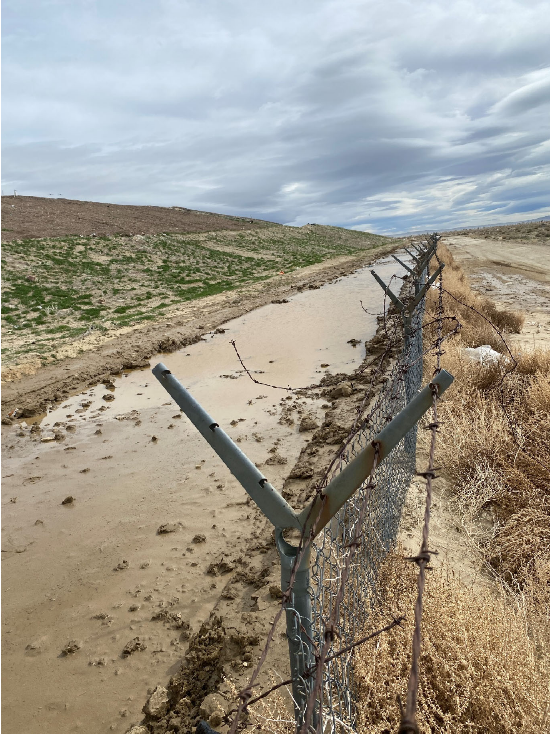
Photo 4: Ponding water, southern perimeter looking east.
