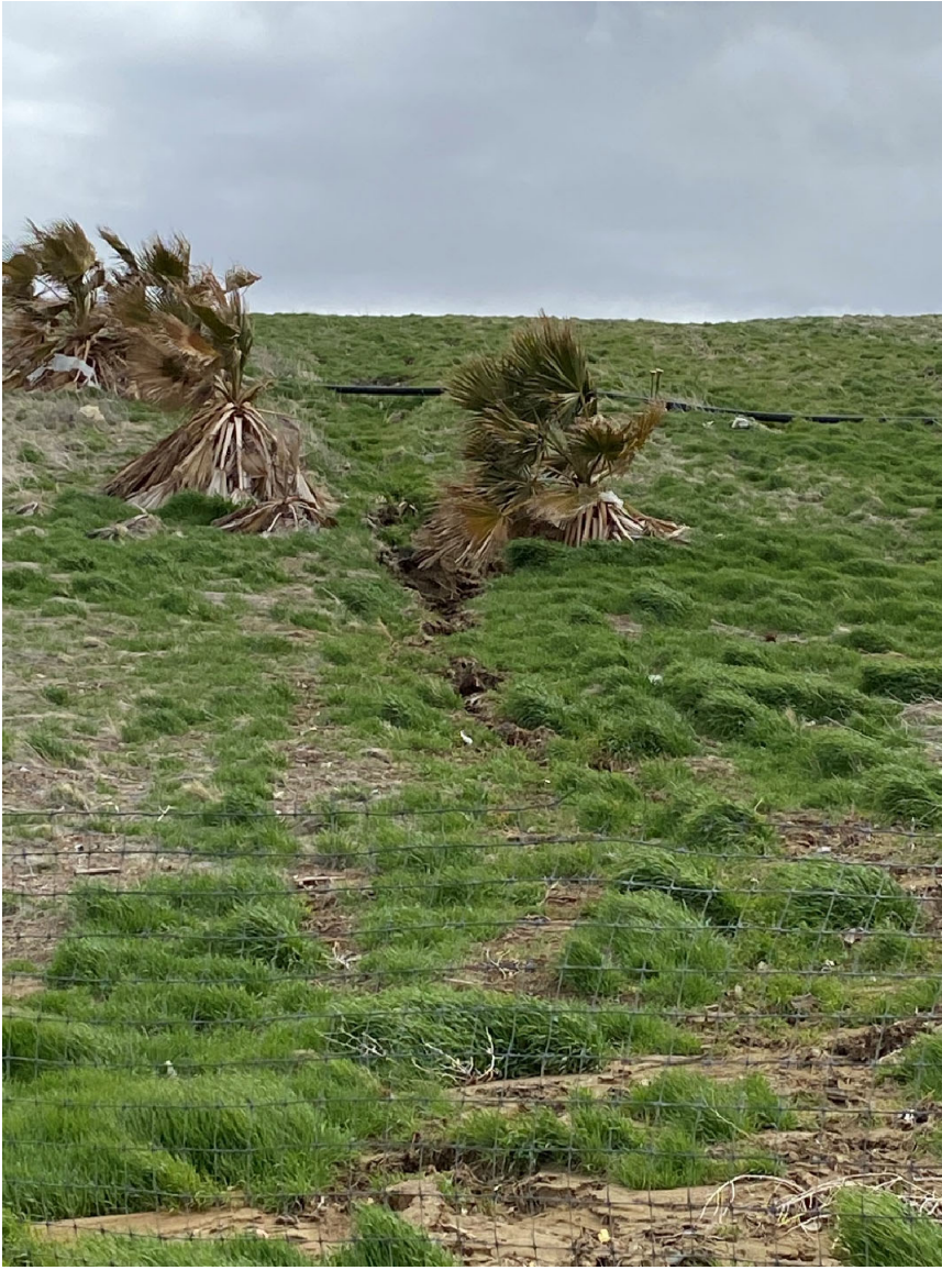
Photo 1: Erosional features between palm trees, northwest portion of landfill.
