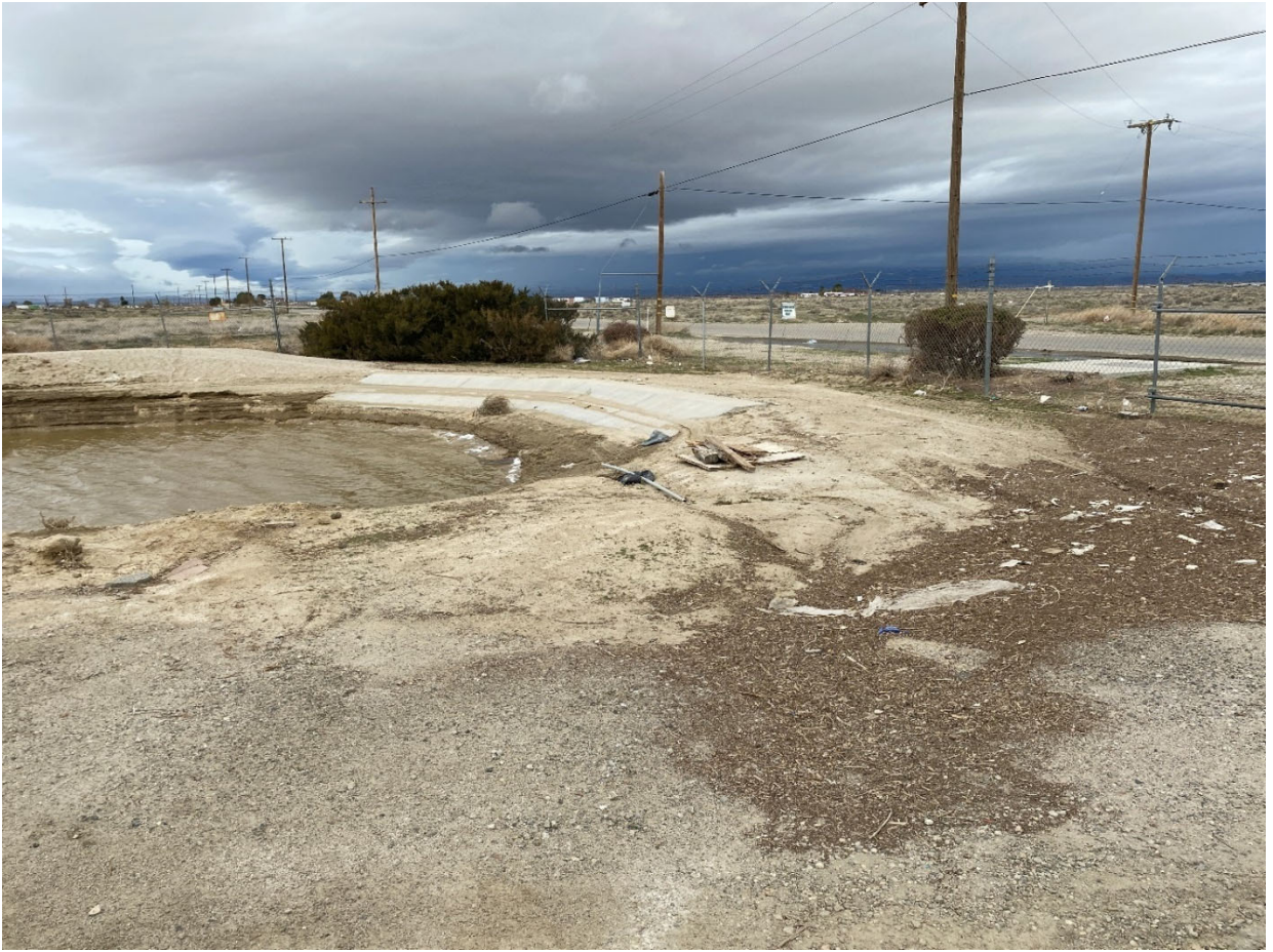
Photo 7: storm water discharge point, overflow by sheet flow.
