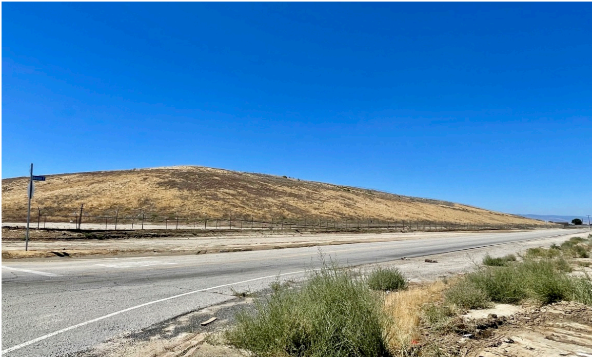
Photograph 4. Looking west from the intersection of Ave F and Challenger Way, at the east end of the north slope.
