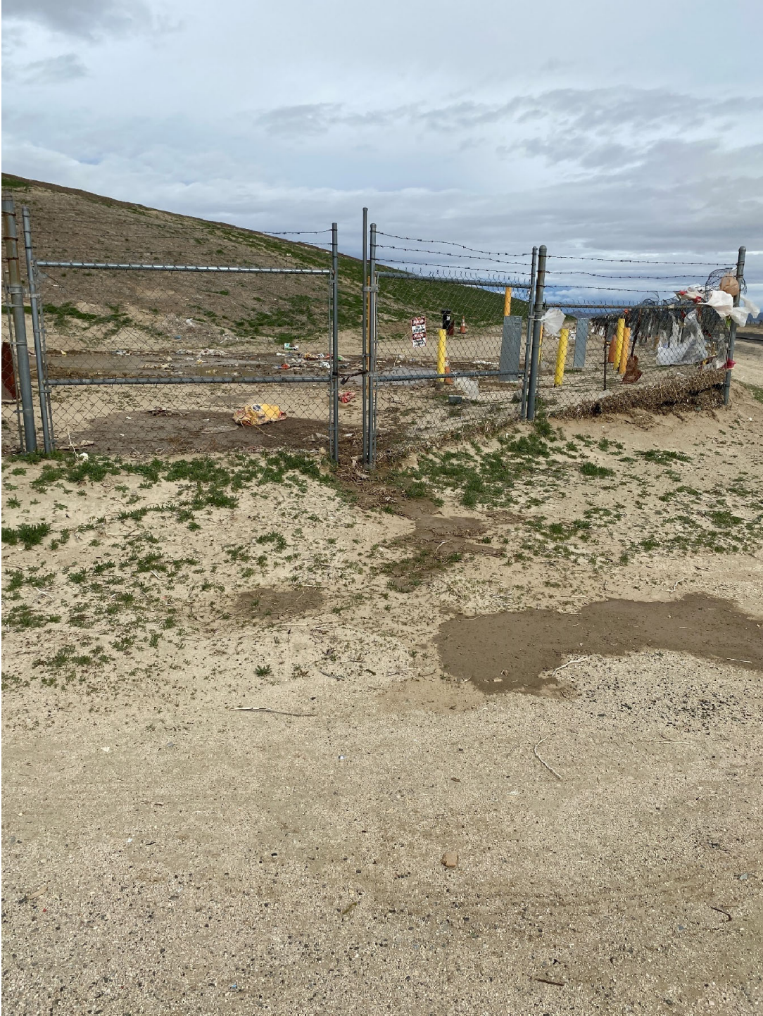
Photo 3: Storm water exiting site at southeast corner of Landfill perimeter.
